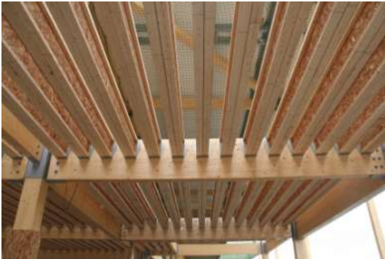
ASDA-Bootle Mezzanine Floor
